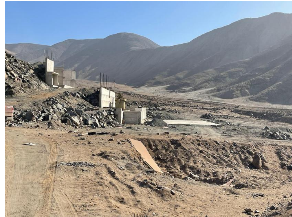
Plant ground works and concrete milling and flotation phase (Nov-25)
