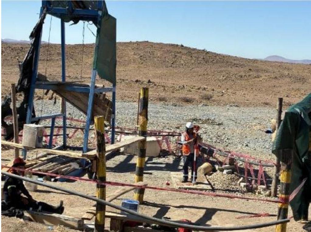
Topographic study covering the Bonanza shaft collar, access path, and first underground platform (Nov-25)
