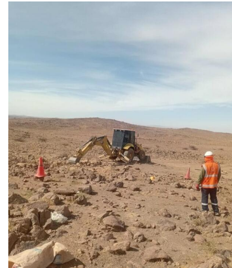
Surface appraisal works including trenches and mapping (Nov-25)
