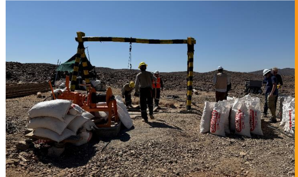
"Bonanza" mine shaft (Aug-24)
